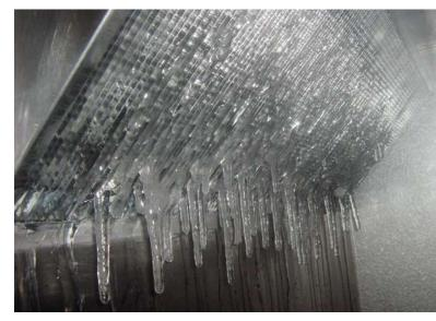
An iced-up energy-recovery system reduces heat-recovery efficiency and increases pressure drops. Effective frost-protection strategies are therefore crucial for efficient operation of an energy-recovery system on cold winter days.
