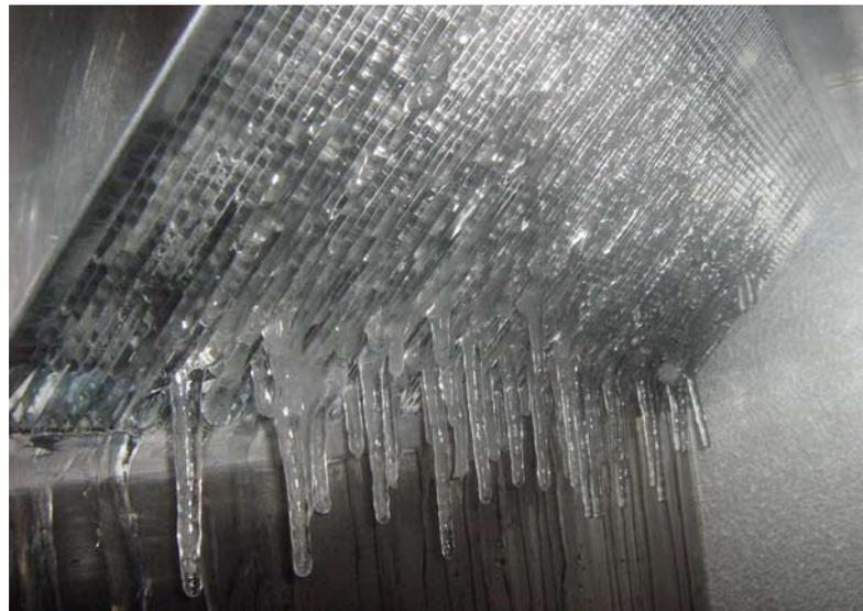
An iced-up energy-recovery system reduces heat-recovery efficiency and increases pressure drops. Effective frost-protection strategies are therefore crucial for efficient operation of an energy-recovery system on cold winter days.
