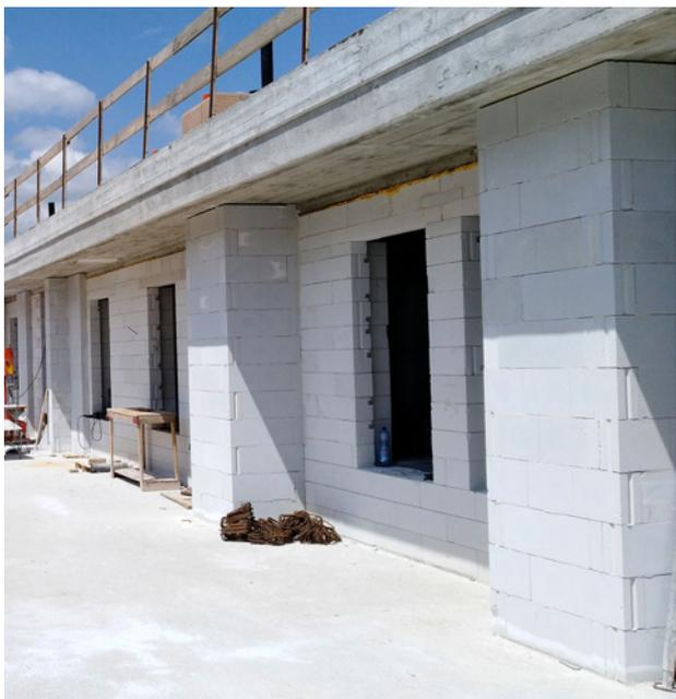
Figure 3. Example of construction works using auto-claved aerated concrete blocks.
