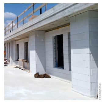
**Figure 3.** Example of construction works using autoclaved aerated concrete blocks.
