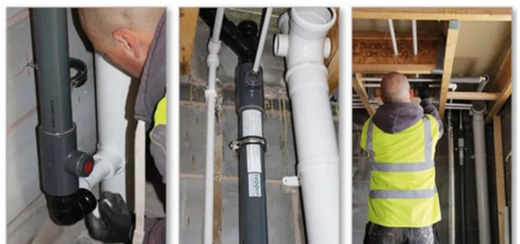
Connecting the Pipe+ HE to the soil pipe
