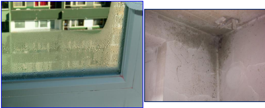
REHVA Apartment after replacement of windows
