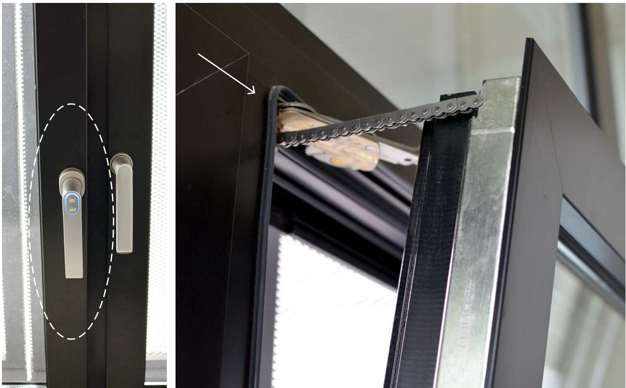
Figure 4. Automated window, with optional manual operation and resistance sensitive gasket.
