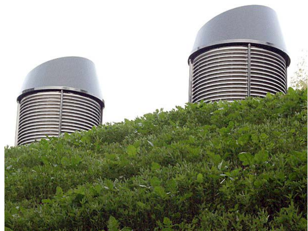
Figure 1. Prefabricated ventilators which utilize the Venturi effect. 3
