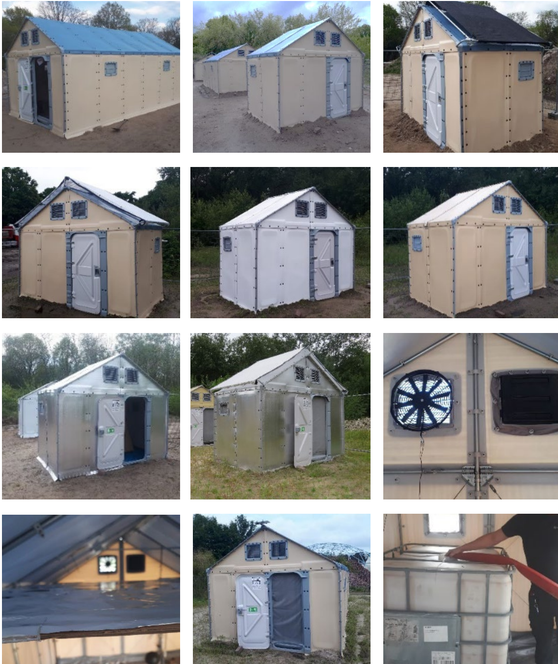
Figure 1. Tested standard RHU and RHUs equipped with overheating countermeasures.
