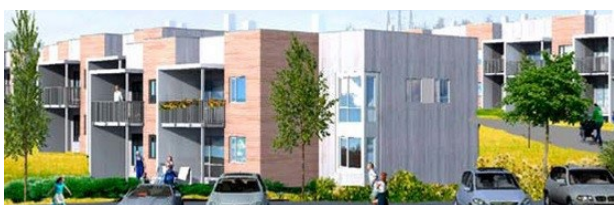
Figure 1. Row low energy house in Trondheim, Norway.
