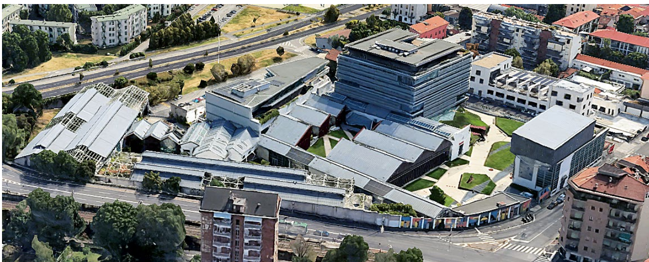
La Forgiatura, Milan – From metal works to carbon-free business park.
