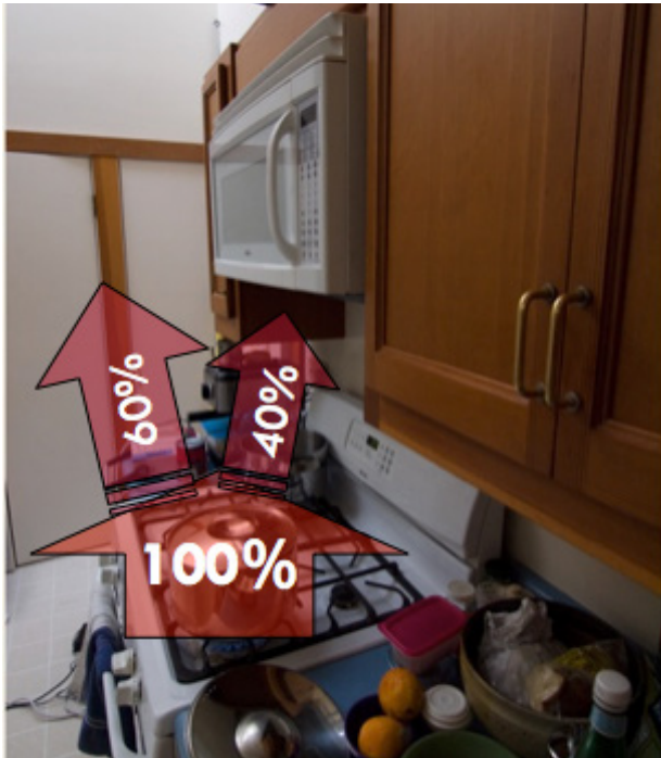
Capture efficiency of a range hood commonly found in the U.S.A (Image courtesy of Iain Walker at the Lawrence Berkeley National Laboratory).
