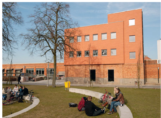
Figure 1. nZEB school building at Technology campus Ghent of KU Leuven (Belgium).
