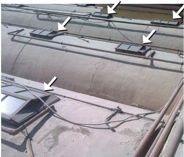
**Figure 4b.** Arrows indicate location of air inlets through naturally openings in the roof.
