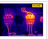
**Figure 2.** The connector to the right shows a higher temperature in all phases because of a higher electrical load.
