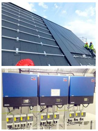
**Figure 3.** Installation of photovoltaic modules on Building B (North Building) and inverters in the AHU room.
