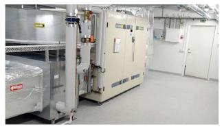
**Figure 2.** The AHU in southern building body, LA1, with supply air duct in the bottom left of the picture with heating coil closest to the ventilation unit and then cooling coil. LA2 in the northern building body is similar.
