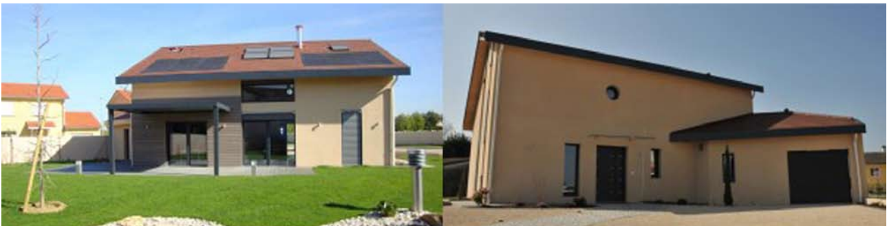
Figure 1. Picture of the Corbioli House, south front (left) and north front (right).
