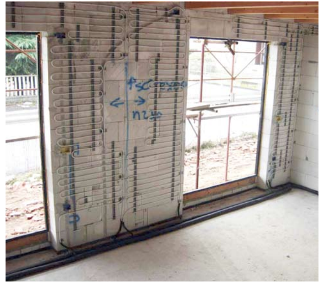
Figure 5. Installation of wall radiant panels.
