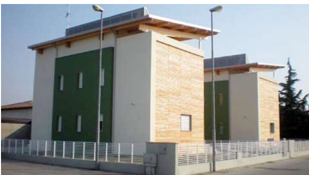
Figure 1. The Eco Sil House , south view.
