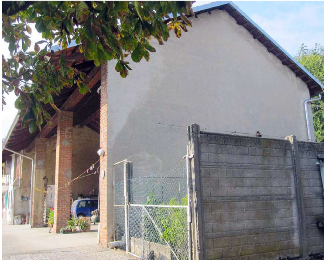
Figure 2. Picture of the pre-existing rural building, south-east side.
