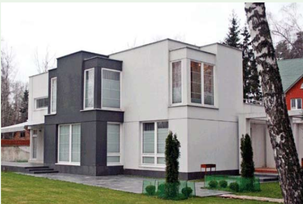
Passive house in South Butovo
