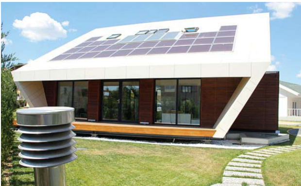
Figure 1. Steelife-EcoHouse South Façade.
