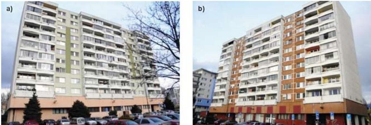
Figure 1. Front sides of the two buildings: a) Before refurbishment b) After refurbishment. [1]
