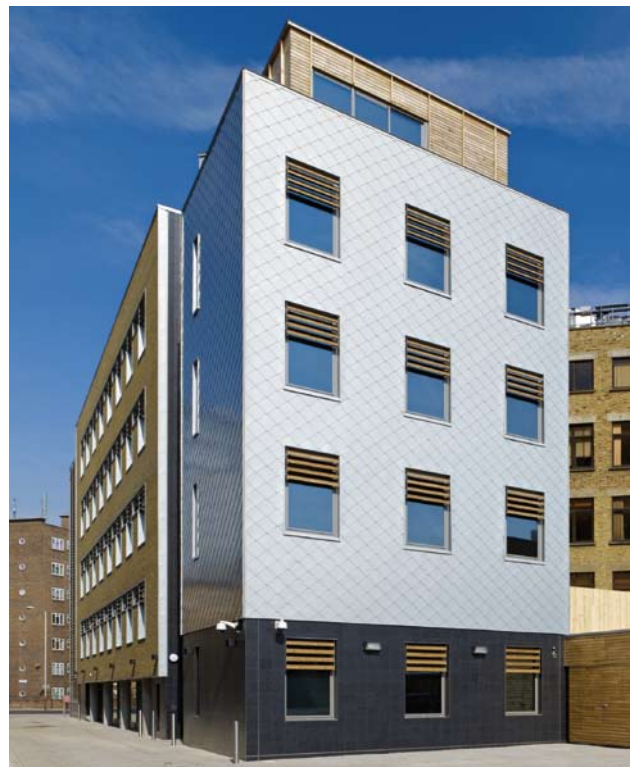
BO CAFOD Headquarters, London, England. Occupying a difficult triangular site, the building is an exemplar of sustainable workplace design with cooling provided by a Thermally Active Building System in the exposed thermal mass in situ concrete structure.
