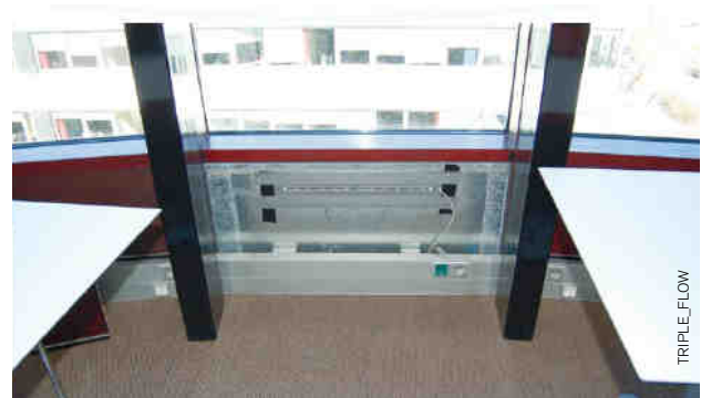
A photo of the façade intake.
