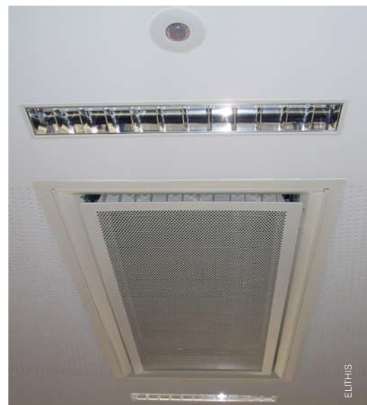
Chilled beams cassettes and lighting installation.
