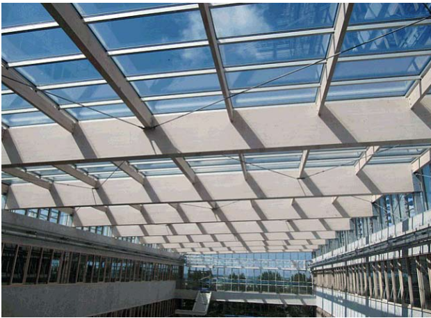
Figure 2. Roof and area of the atrium.
