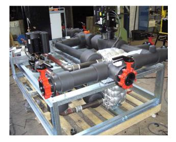
Figure 9. BHE/solar array control unit during its construction.
