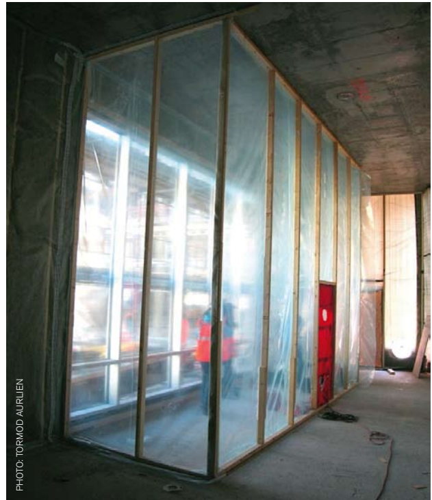
Figure 1. Temporary “tent” made from plastic foil, with a (red) blower door mounted. The amount of air that is sucked out of the tent by the fan in the blower door equals the leaking air that pass through the details of the façade being tested. A person inside the tent may easily detect air-leakages in the façade by just feeling with his hand along joints and details in question, if the air pressure inside the tent is kept at a lower level than the outside (around 50 Pa). This picture is from a new large building with passive-house ambition ( n_{50} < 0.6 \text{ h}^{-1} ).
