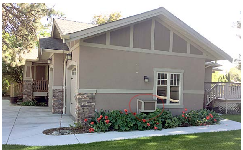
Figure 4. Outdoor air inlet box and filter housing (circled) – case study house.
