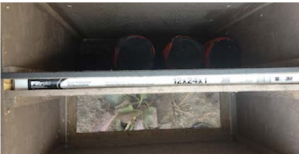
Figure 5. Air inlet with screen, mesh and filter – all upstream of the earth tubes.
