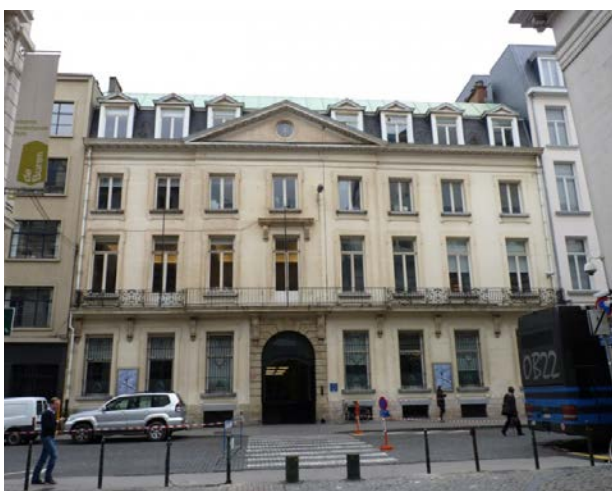
Figure 2. Technical building façade at 23, rue Léopold.
