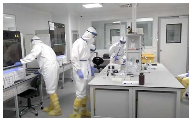
Figure 5. Laboratory in Nis in equipment installation phase.
