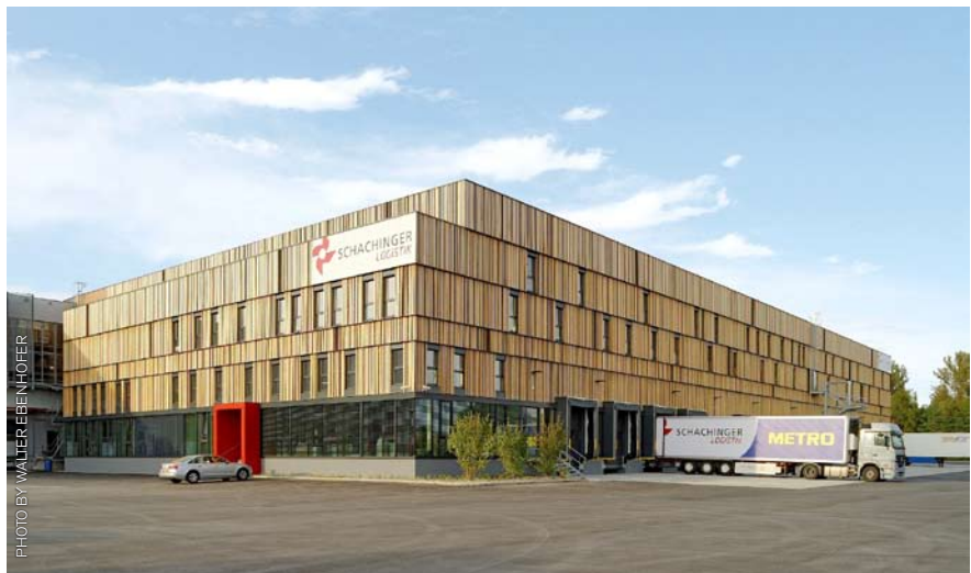
Main entrance of the office wing and delivery area.
