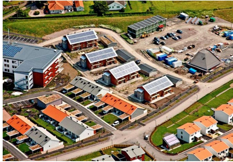
Figure 1. Passive house residential area Vallda Heberg during construction [4].
