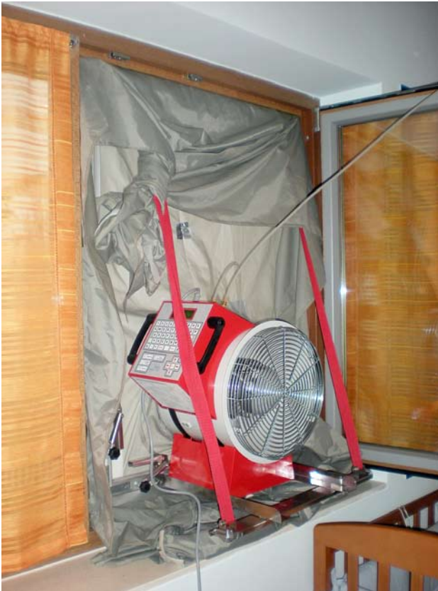
Figure 4. Blower Door test.
