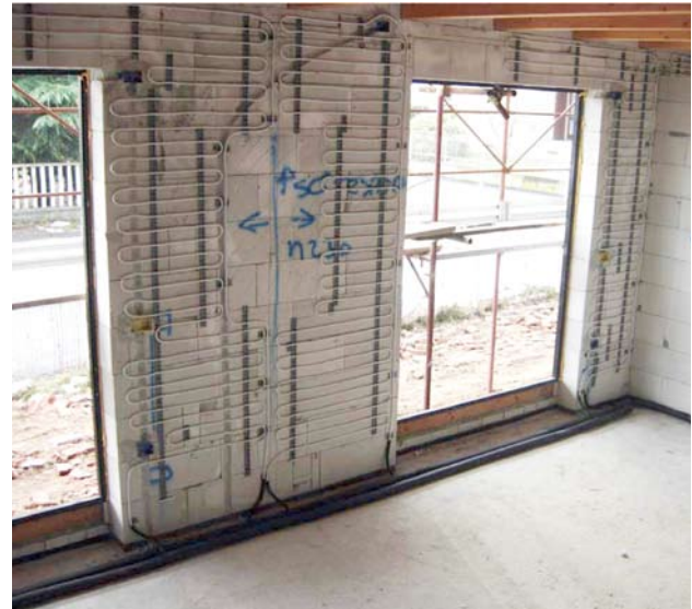
Figure 5. Installation of wall radiant panels.
