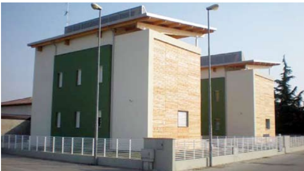
Figure 1. The Eco Sil House , south view.
