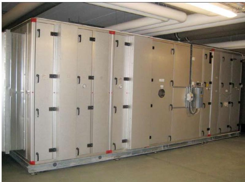
**Figure 4.** Low Speed Air Handling Unit without sound attenuators. The air flow is 13 m<sup>3</sup>/s. The speed through the AHU is 1.6 m/s.
