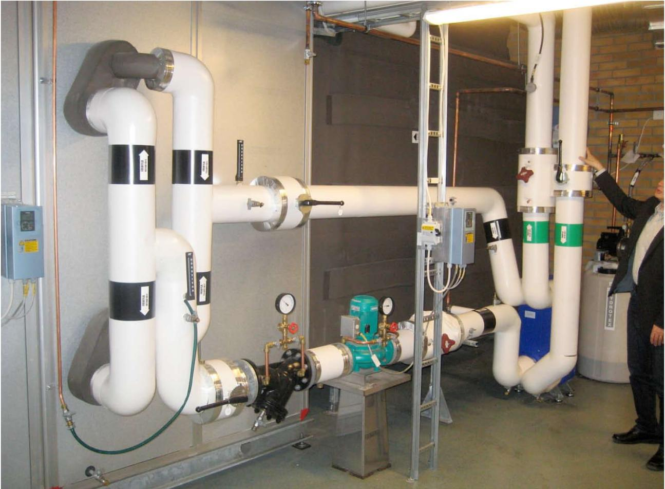
**Figure 3.** Free cooling coil as first step in the AHU. From the right: the heat exchanger that exchanges the heat from the glycol circuit in the coil in the AHU to the chilled water circuit for cooling beam system. Energy saving is approx 5 – 10 kWh/m<sup>2</sup> annually.
