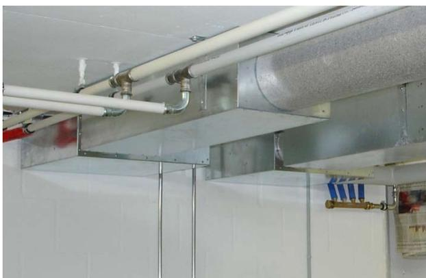
**Figure 2.** Two blue mounting plates (top) are nailed to the wooden formwork and connected to the ComfoTube ducts, later covered by liquid concrete. Once the formwork is dismantled, the distribution casings can be bolted to the mounting plates, then visible on the ceiling. Below right both the distribution casings for fresh and return air can be seen, connected to the sound absorbers in front of them.
