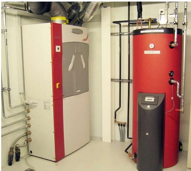
**Figure 4.** Comfortable energy efficient homes often are equipped with standardized combined units: A Zehnder ComfoBox provides not only heat recovery ventilation to the building on the left, but also space heating, space cooling and domestic hot water by an energy efficient soil to water heat pump, reducing cost for planning and installation.
