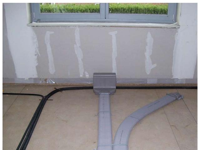
**Figure 3.** Each country has its own construction principles. Whereas in Switzerland and Austria most concrete ceilings are poured on site onto site built wooden formwork, in which round ComfoTube ducts can be mounted, prefab hollow ceiling-elements are applied in Northern Germany, on which flat ComfoTubes are positioned in the layer of the impact noise insulation.
