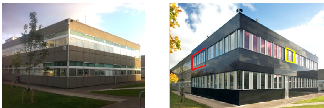
Figure 1. External facades; existing 1974 building (left) and retrofitted zero2020 test-bed building (right) where red indicates the location of the thermal comfort study and yellow indicates the location of the ventilation rate performance experiments.
