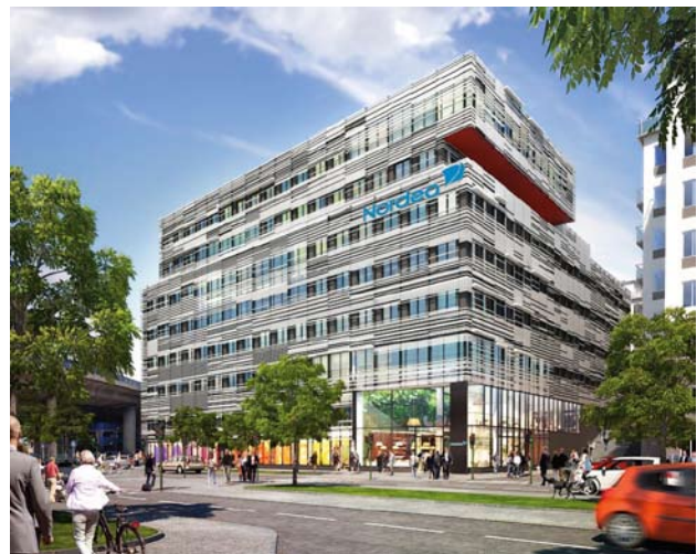
Figure 1. The façade with external sun shading.
