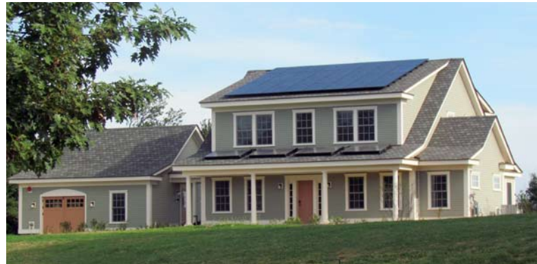
Net Zero Energy Research Test Facility (NZERTF) at NIST.
