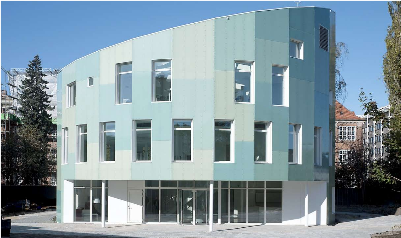
Figure 2. An example of a NZEB in Denmark, Green Lighthouse. It was built in less than a year in a close public/private partnership. The partners are the University of Copenhagen, VELUX, VELFAC, the Danish Building and Property Agency (UBST) and the City of Copenhagen. Green Lighthouse is located at the Faculty of Science at the University of Copenhagen and is a one-stop-shop where students can get advice on their studies, exams etc. (Photo: greenlighthouse.ku.dk)
