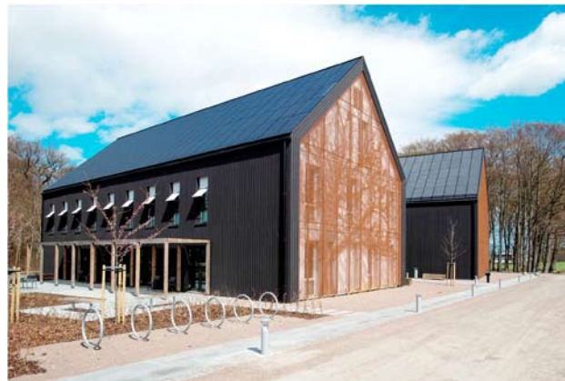
Figure 1. Left: Orientation of building. Right: Photo taken from the south. The overall design concept for energy efficiency follows the passive house design principle with a highly insulated and airtight building envelope and a balanced ventilation system with high heat recovery. Heat is produced by a geothermal heat pump and free-cooling is extracted from the bore holes during summer. Roof sides facing south west are equipped with PV panels. A summary of the building constructions is presented in Table 1 .
