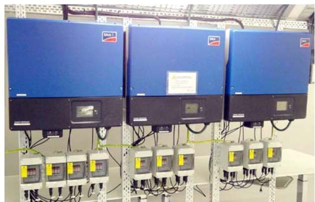
Figure 3. Installation of photovoltaic modules on Building B (North Building) and inverters in the AHU room.
