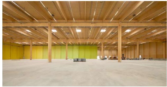
Interior of the warehouse with a detailed view of the wood structure.
