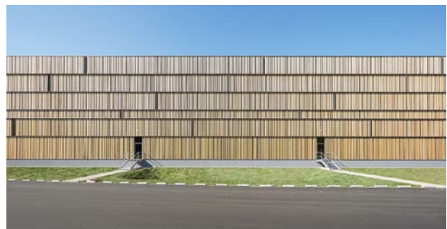
East façade with its barcode-like appearance.
