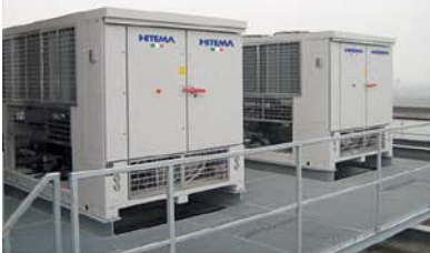
Inverter Technology Compressors - Total Load 3,2 Mw
