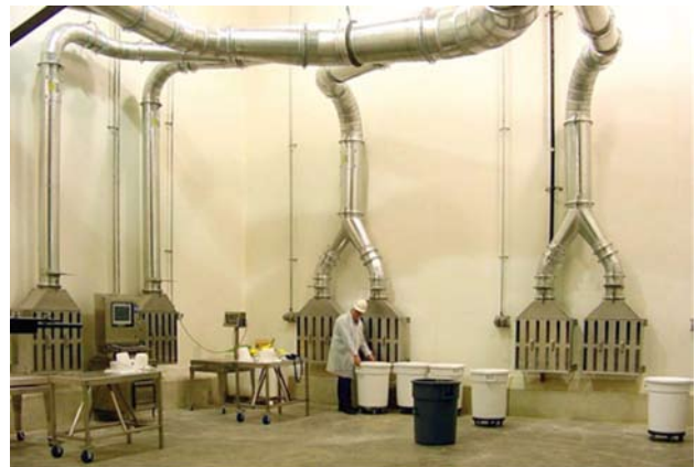
Figure 1. Typical hood system.
