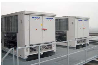
Inverter Technology Compressors - Total Load 3,2 Mw
