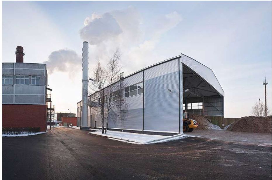
Figure 2. The biofuel fired boiler house at the plant Vecmilgravis.
