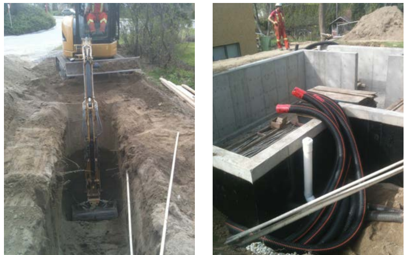
Figure 3. Trenching and laying earth tubes for case study project.
