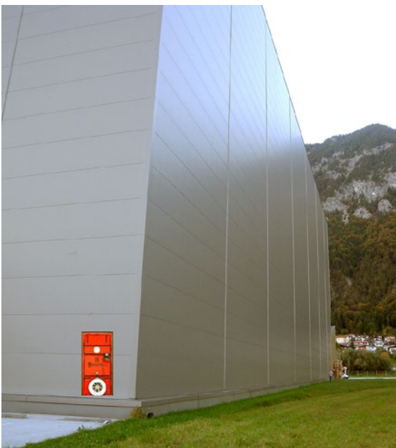
Figure 1. Warehouse for herbs with an air change rate n_{50} = 0.03 \text{ h}^{-1} , internal Volume V = 46,400 \text{ m}^3 and airflow at 50 Pa V_{50} = 1.620 \text{ m}^3/\text{h} .
