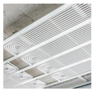
**Figure 2.** Uponor Thermatop M is a suspended radiant heating and cooling ceiling system that consists of diffusion-resistant multilayer composite pipes. It is mounted on conventional ceiling substructures.
