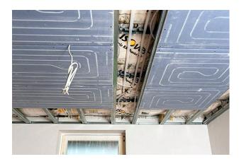
**Figure 3.** Uponor Renovis is a drywall system in which piping has been pre-installed at the factory. The elements can be mounted on virtually all wall substrates. This makes Renovis also ideal for renovation projects.
