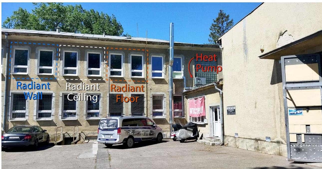
**Figure 1.** Office building with laboratory for testing radiant systems. (Author: Martin Šimko)
