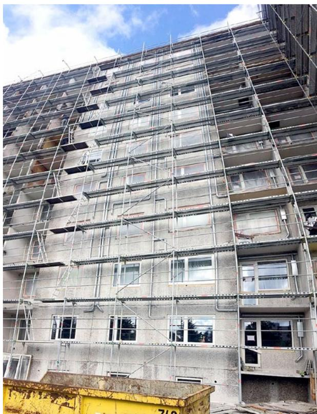
**Figure 2.** Estonian apartment building renovated with KredEx grant (30% of financial support) that requires to install heat recovery ventilation. On the photo, ventilation supply air ductwork and some parts of extract ductwork are installed on the façade before additional insulation, and heat recovery ventilation unit will be installed to the renovated roof.
